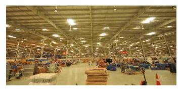
"Steel is used in the PEB structures. All the primary members are fabricated out of high strength steel plates with minimum yield strength of 345 mpa. While the secondary members such as purlins are manufactured out of galvanised steel with higher galvanised coating of 275 gsm and yield strength of 345 mpa. Roofing sheets are manufactured of Bare Alu Zinc with yield strength of 550 mpa,
